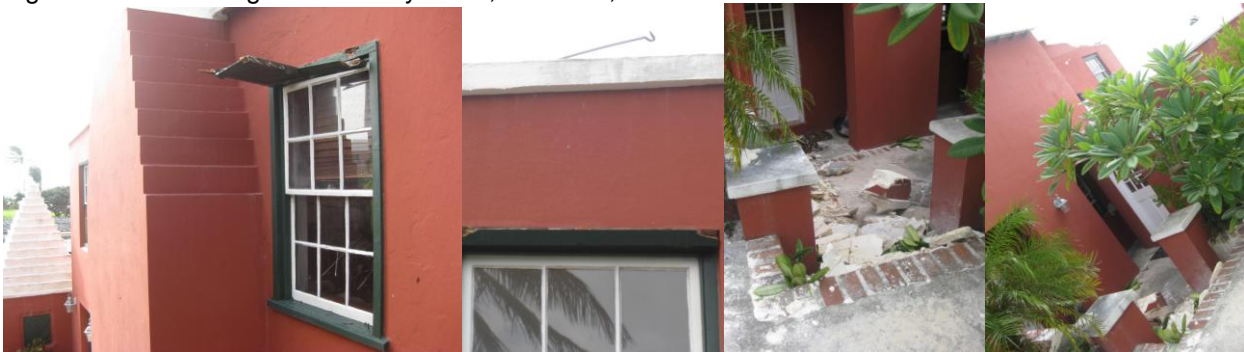
Figure 5: Evidence of rotation: torn blinds on the lee side of Pitts Bay Rd House, Blind hook found on TOP of house (behind and above original location), chunks of roof found 20ft SW of origin
